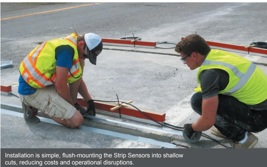
Installation is simple, flush-mounting the Strip Sensors into shallow cuts, reducing costs and operational disruptions.
